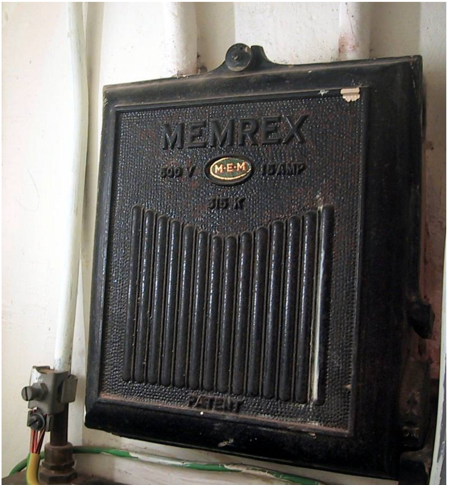
This Cast Iron fusebox was found in a property, built in 1932.
